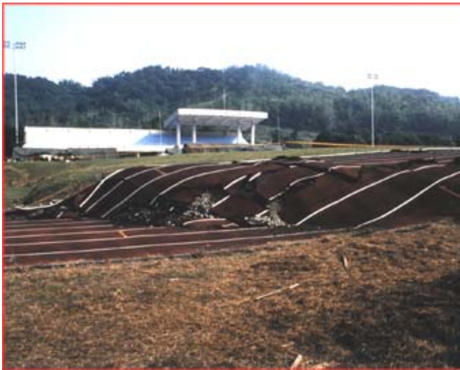
Figure 12 Photograph taken of a surface rupture related to the 1999 Chi-Chi earthquake, Taiwan. The view is looking toward the fault, which has ruptured through a school's 400 m athletic track, which was obviously flat before the rupture. Note how the scarp has grown by thrusting out and over the former ground surface, and how deformation is focused in the hangingwall (uplifted) block.
